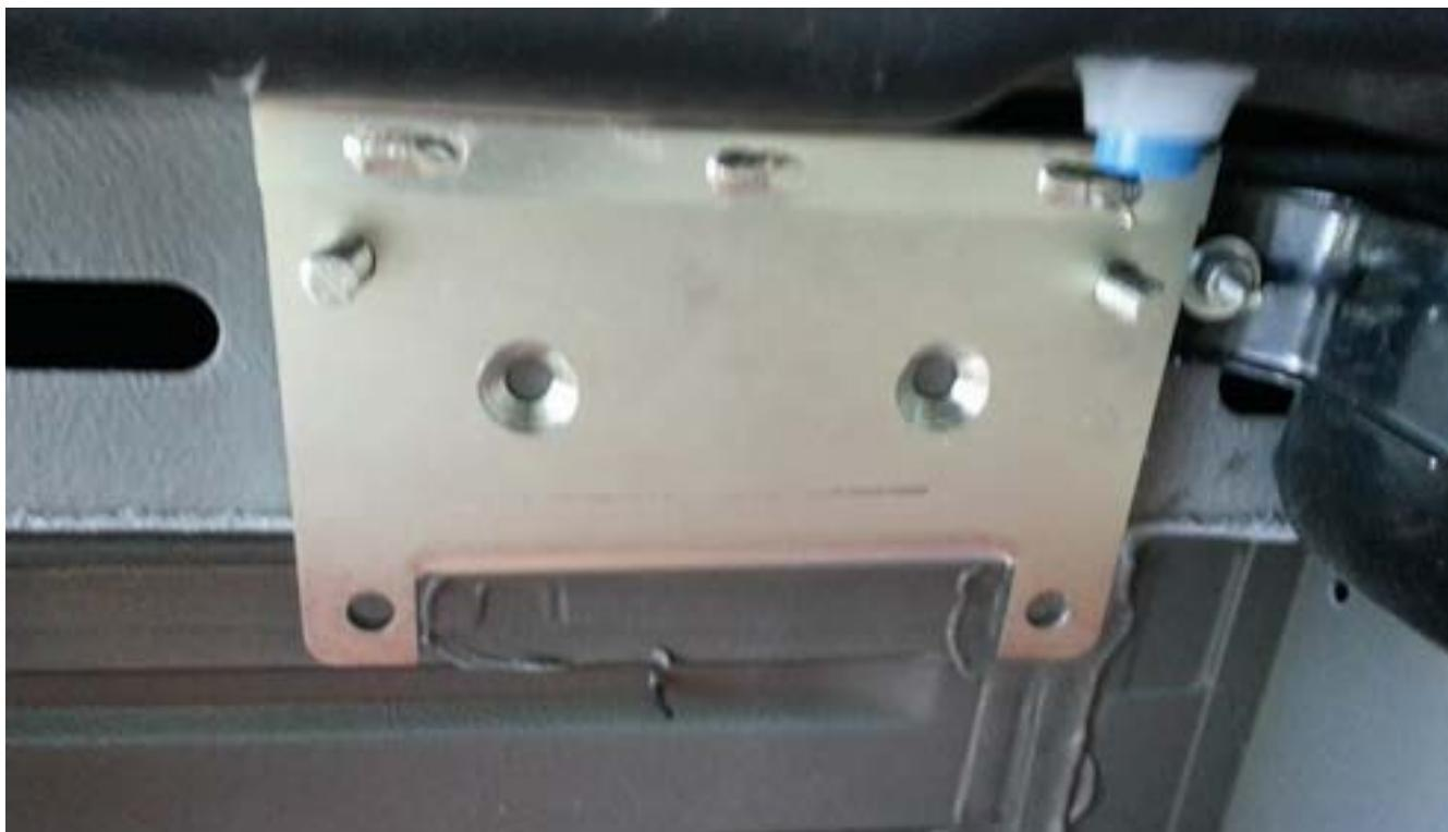
Drill two 10 mm holes following the templet formed by the support, as shown in the photo.
